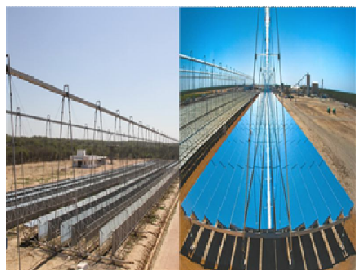
Fig. 5: Linear Fresnel Reflector (LFR)
